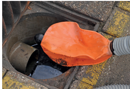
Attach the ROM SmokeStopper at the end of the smoke supply hose
