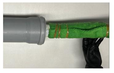
Insert the prepared Packer into the pipe.
