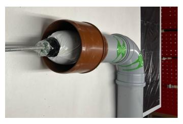
Keep Packer pressurised until patch is cured completely. Resin curing time depends of type of the resin that is used and the temperature. Curing takes longer in a cold environment.
