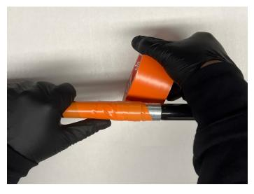
Wrap protective tape around each fitting to prevent resin from getting inside fittings.
