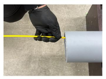
Carefully push the camera through the pipe until the camera head is in the centre of the damaged section of pipe where the repair is to be installed.
