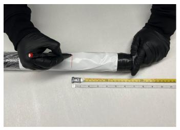
Copy the off-limit-zone measure on to the surface of the support hose using a marker pen.
