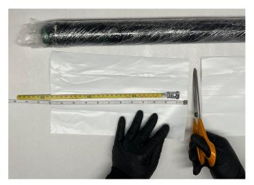
When using support only on the ends, the hose should be measured in way it will reach at **minimum 10cm (4")** under the patch. The same rule applies when patches are shorter than the full length.
