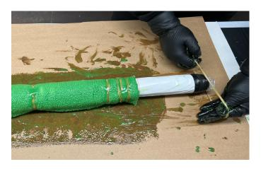
After the end caps side has been secured, start applying rubber bands every 10-15cm (4"-5").
